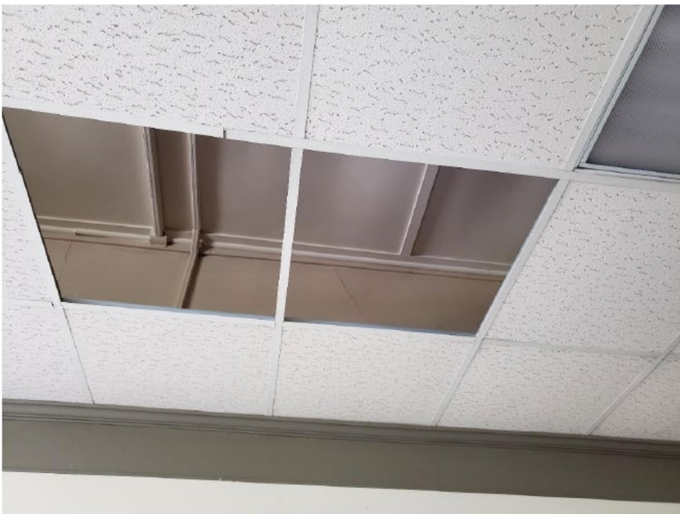
Photo 8: First Floor Reinforced Ceiling Above Hung Acoustical Ceiling
