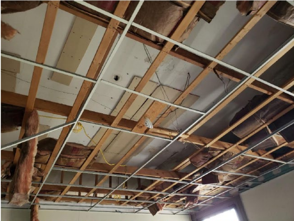
Photo 9: Second Level Ceiling Attached to Attic Framing
